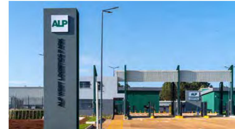
Ground floor offices open directly onto the warehouse floor
